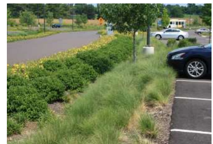
Einstein infiltration trench (Foto: Montgomery County Planning Commission)
