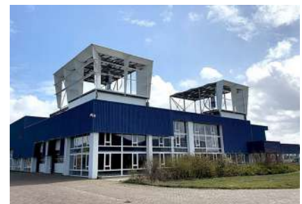
PowerNEST-installatie in Katwijk (Foto: IbisPower)
