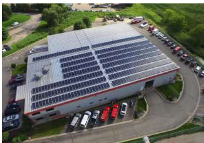
Dave Jones Plumbing, Madison, WI (Foto: US Department of Energy)
